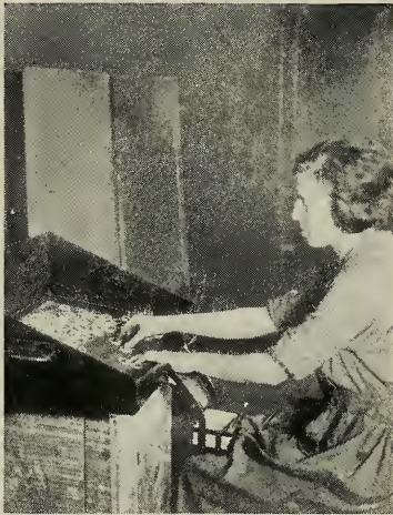
PARTS ARE COUNTED BY "FIVE'S" The small carton in the rack must be filled with exactly 100 of the small parts. See page 121 for item
